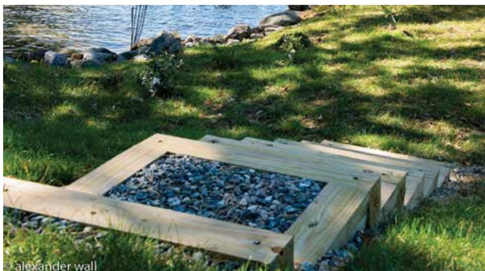
Figure 2. Infiltration steps recommended during a LakeSmart evaluation and installed at a shoreline property to slow the flow of nutrient laden runoff into an adjacent lake.
